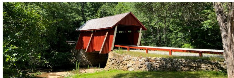
Campbells Covered Bridge © Greenville County
