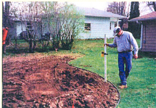
The rain garden is dug to 3 to 4 inches in depth with care to make the bottom as level as possible. With the lawn sloping gently upward to the house, the garden is positioned to trap water from a downspout.
