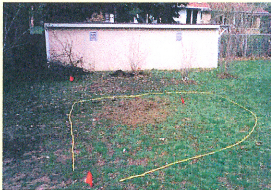
Rope is used to lay out the boundary of a future rain garden.
