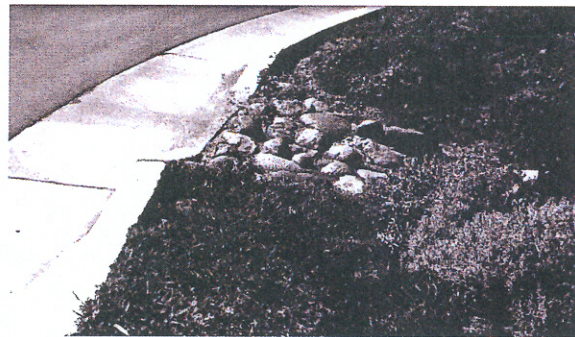
Inlet detail for urban curb/swale system
