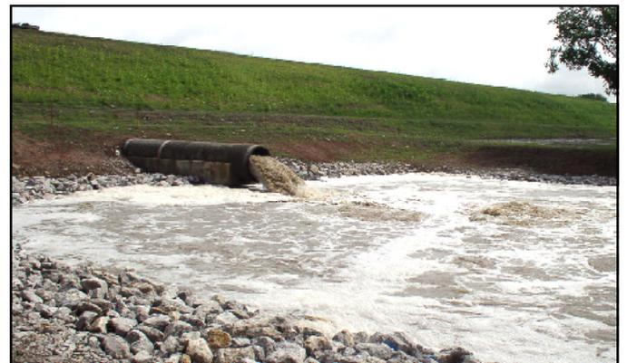
Water is released through a pipe in the dam for several days after a heavy rainstorm.
