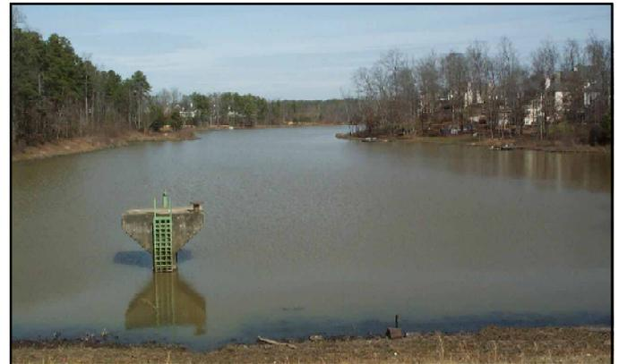
A concrete inlet tower (might be metal on older dams) connected to a pipe extending through the dam serves as a principal spillway for dams, controlling the water level. A slide gate at the bottom of the inlet can be opened to lower the water level for maintenance and repair.
