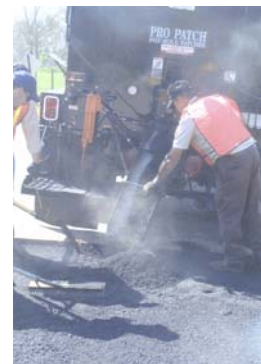
Road Crews Working
