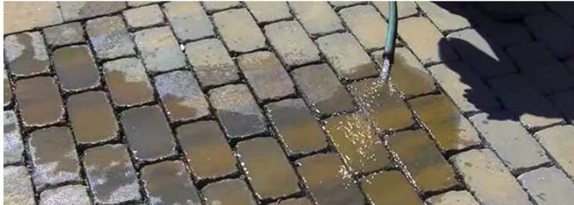
or grid concrete pavers underlain by a drainage layer. A permeable paver system allows stormwater runoff to pass in between the paver surface and into an underlying stone reservoir, where it is temporarily stored and allowed to infiltrate into the underlying soils. When properly sized, installed, and maintained, permeable pavers may provide reductions in stormwater runoff and pollutant loads.
