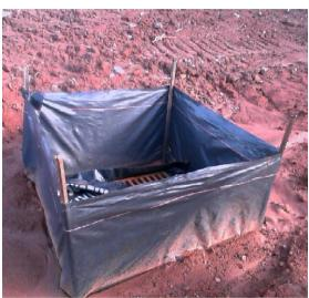
SC-07A Type A Inlet Protection – Filter Fabric
