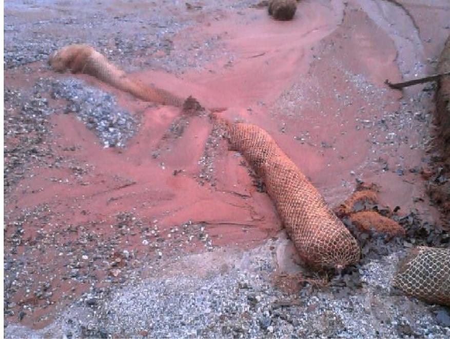
SC-05 Sediment Tube Ditch Check
