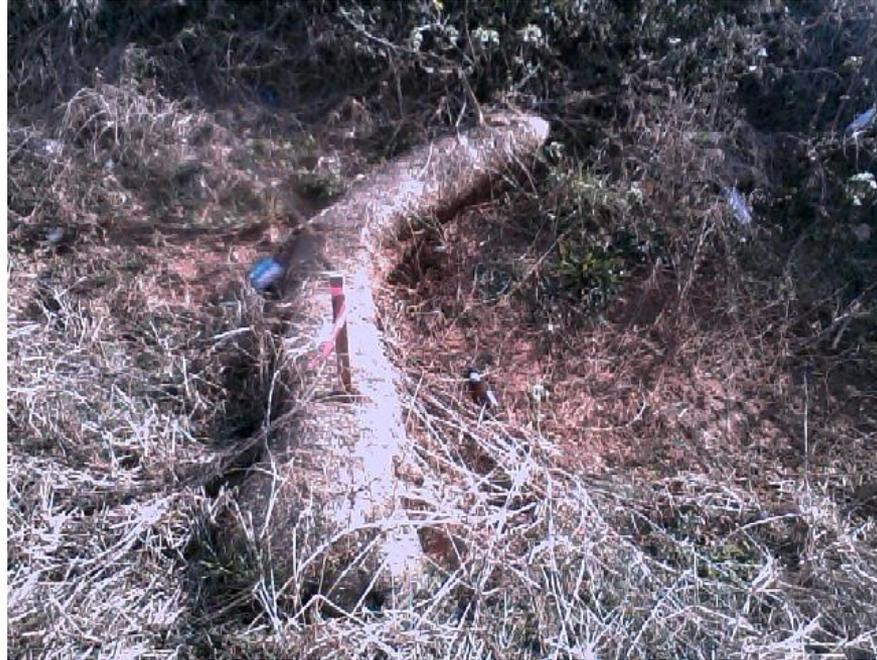
SC-05 Sediment Tube Ditch Check
