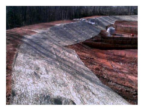
**EC-04 Rolled Erosion Control Products**
