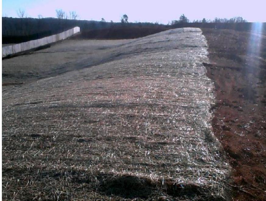
EC-04 Rolled Erosion Control Products
