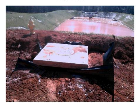
SC-07A Type A Inlet Protection – Filter Fabric
