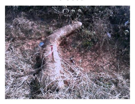
SC-05 Sediment Tube Ditch Check
