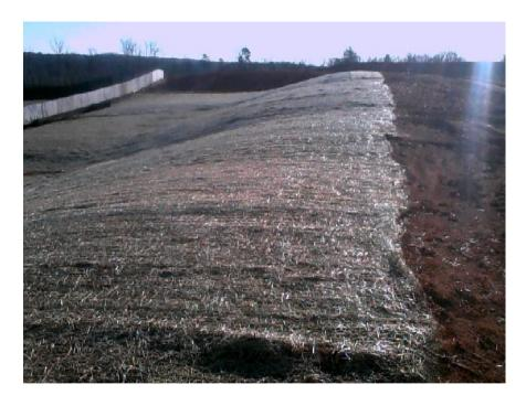
**EC-04 Rolled Erosion Control Products**
