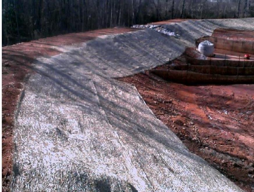
EC-04 Rolled Erosion Control Products
