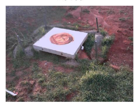
SC-07A Type A Inlet Filter – Sediment Tube
