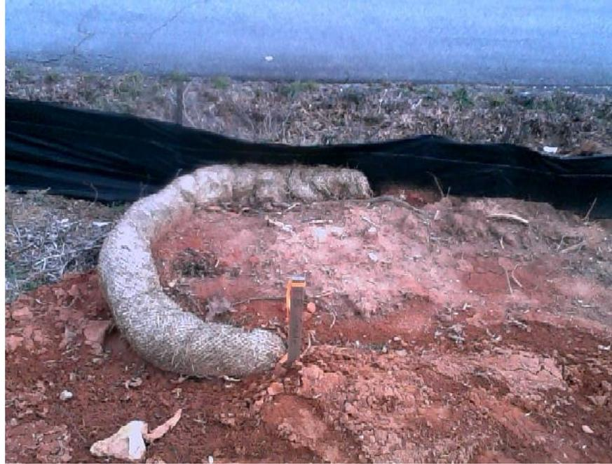
SC-05 Sediment Tube Ditch Check
