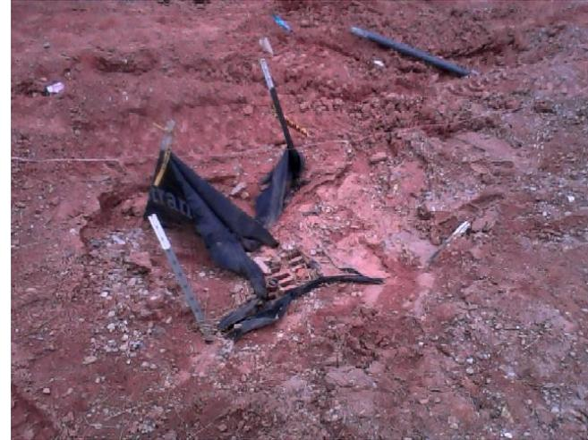
SC-07A Type A Inlet Protection – Filter Fabric
