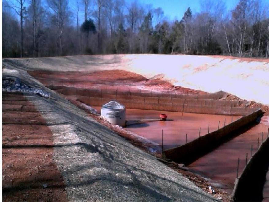
SC-01 Surface Outlet and Baffle Sediment Basin
