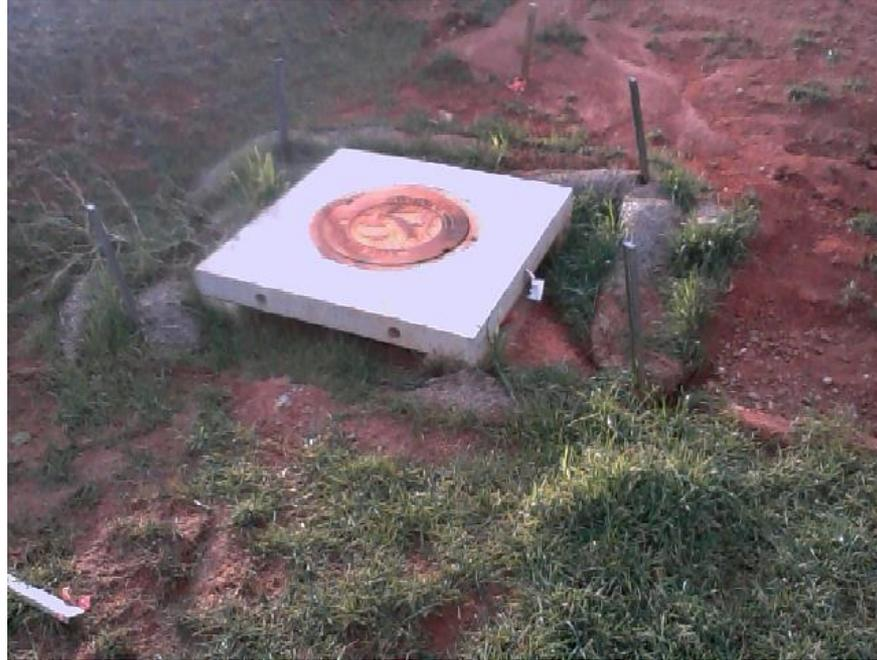
SC-07A Type A Inlet Filter – Sediment Tube
