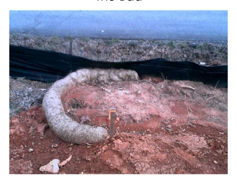
SC-05 Sediment Tube Ditch Check
