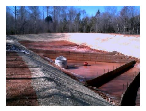
SC-01 Surface Outlet and Baffle Sediment Basin
