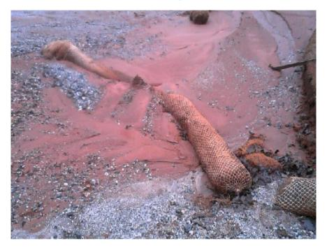
SC-05 Sediment Tube Ditch Check
