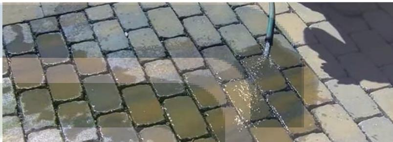
or grid concrete pavers underlain by a drainage layer. A permeable paver system allows stormwater runoff to pass in between the paver surface and into an underlying stone reservoir, where it is temporarily stored and allowed to infiltrate into the underlying soils. When properly sized, installed, and maintained, permeable pavers may provide reductions in stormwater runoff and pollutant loads.
