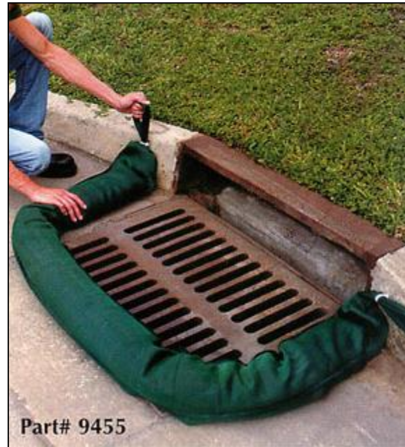
Proper inlet protection for catch basins
