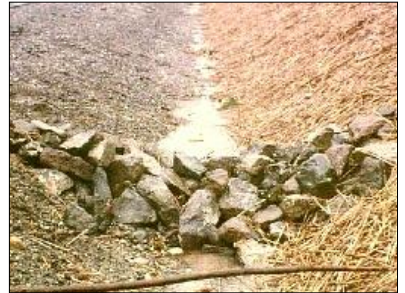
Rolled erosion control products and natural or manufactured ditch checks to slow down runoff and trap sediment
