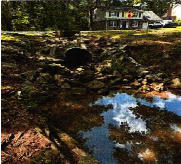
Culvert under Paddock Drive
