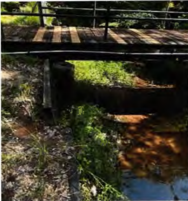
Bridge and Bulkhead
