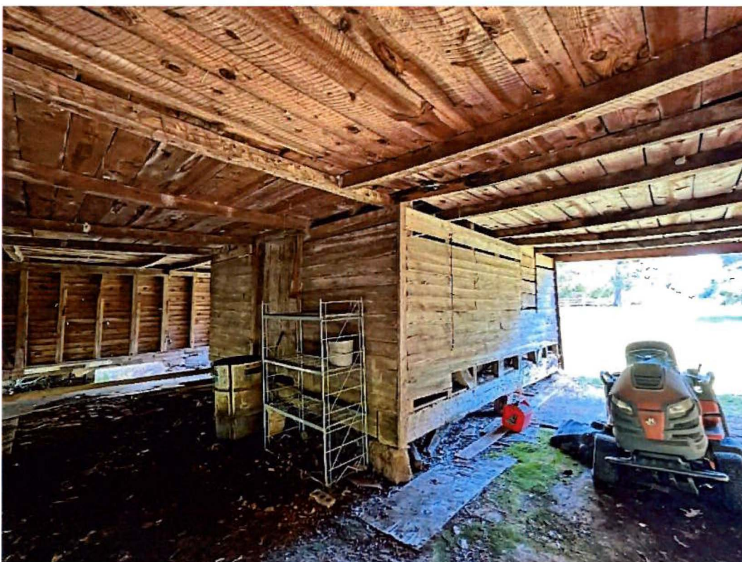
Image 20: slave cabin inside barn; siding gaps, wood window infill top right, missing sill
