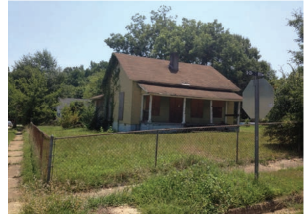
An old mill house awaits repair or demolition
