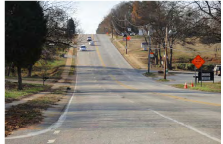
Four-lane section of Conestee Rd.
