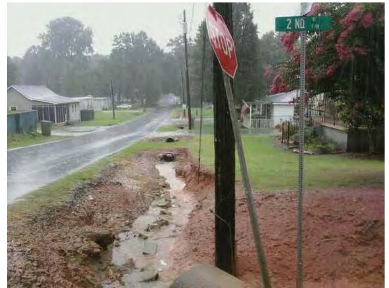
Improved drainage at intersection of 2nd St. and 3rd Ave.
