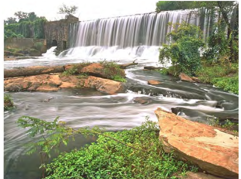
Historic Lake Conestee Dam and Spillway Courtesy: Ben Keys
