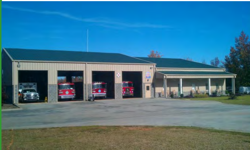
Belmont Fire Department, 701 Fork Shoals Road, Conestee, SC Courtesy: Belmont Fire Department
