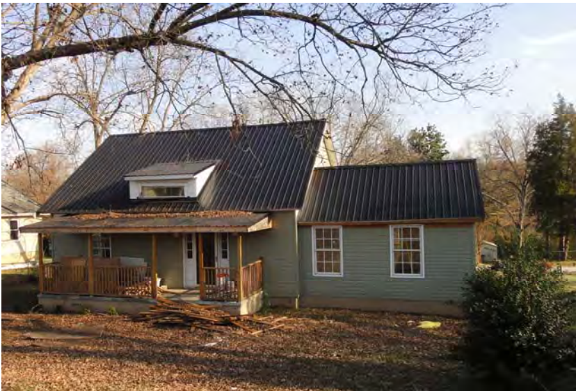
Renovation of house along 3rd Avenue
