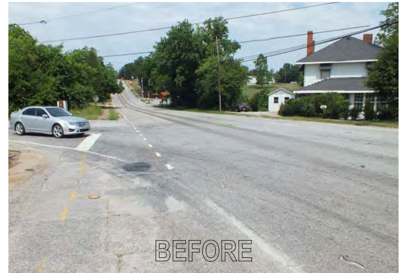
Current view of four-lane section of Conestee Rd. from Main St.
