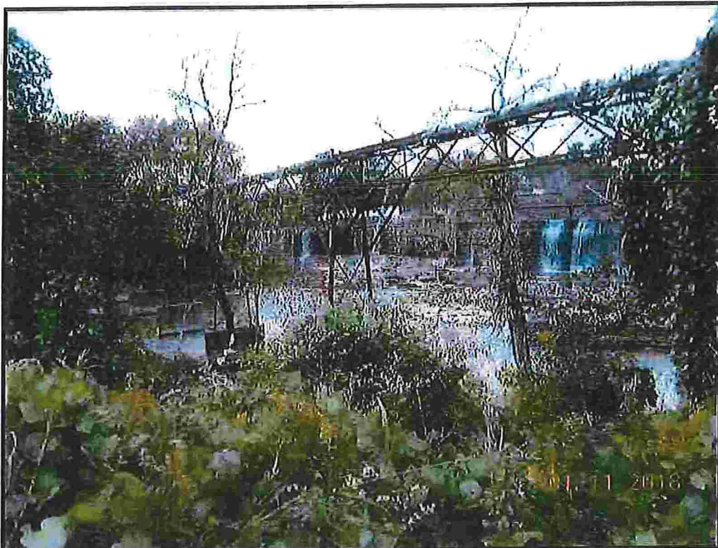
Photo 10: Pipeline crossing the Saluda River along the western property boundary.
