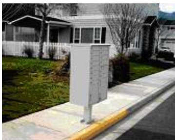
INCORRECT - THE ADA REQUIRES THAT SIDEWALKS REMAIN CLEAR
