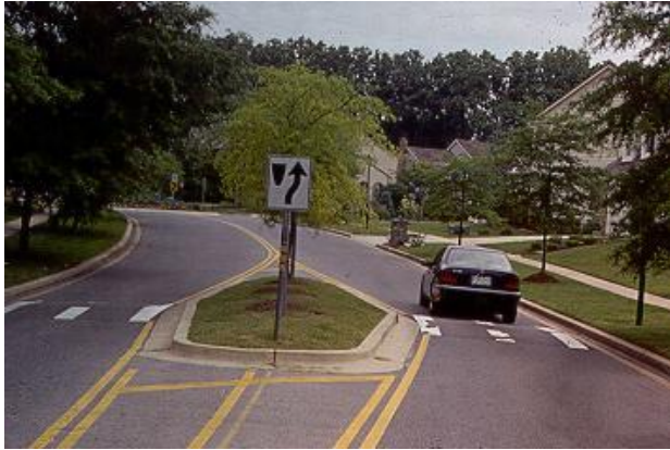
Raised Crosswalk with Center Island
