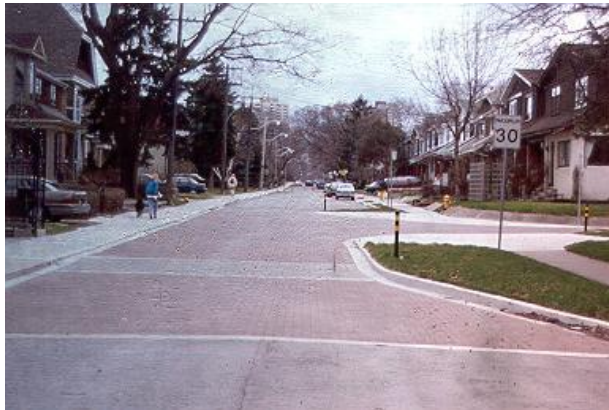
Raised Intersection with Neckdown
