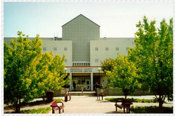
Greenville County Detention Center
