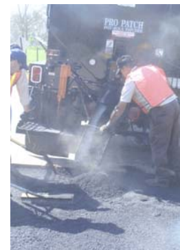
Road Crews Working
