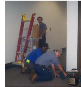
Carpet Repair at County Square
