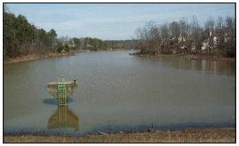
A concrete inlet tower (might be metal on older dams) connected to a pipe extending through the dam serves as a principal spillway for dams, controlling the water level. A slide gate at the bottom of the inlet can be opened to lower the water level for maintenance and repair.
