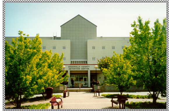
Greenville County Detention Center
