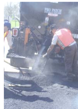
Road Crews Working
